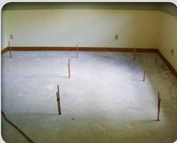
Indoor urethane injection installation.
