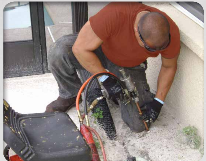
Outdoor urethane injection installation.
